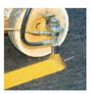
Product Description Synthetic resin based, cold road line paint with solvent.
