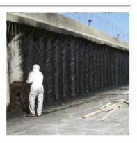
Product Description Teknofast is water based, fast setting polymer modified bitumen waterproofing material.
