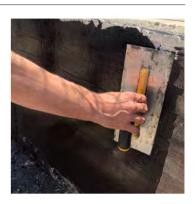
Product Description Teknoflex is waterproofing material that polymer modyfied bitumen based, resistance to enviromental condition.
