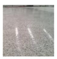
Product Description TEKNOSER LITYUM is a low viscosity lithium silicate based liquid surface hardener.
